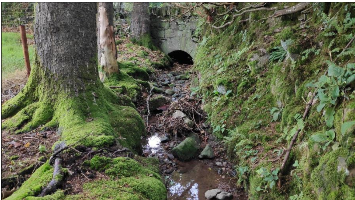
Plate 3.15 Representative image of site C1 on an unnamed stream, September 2020.
